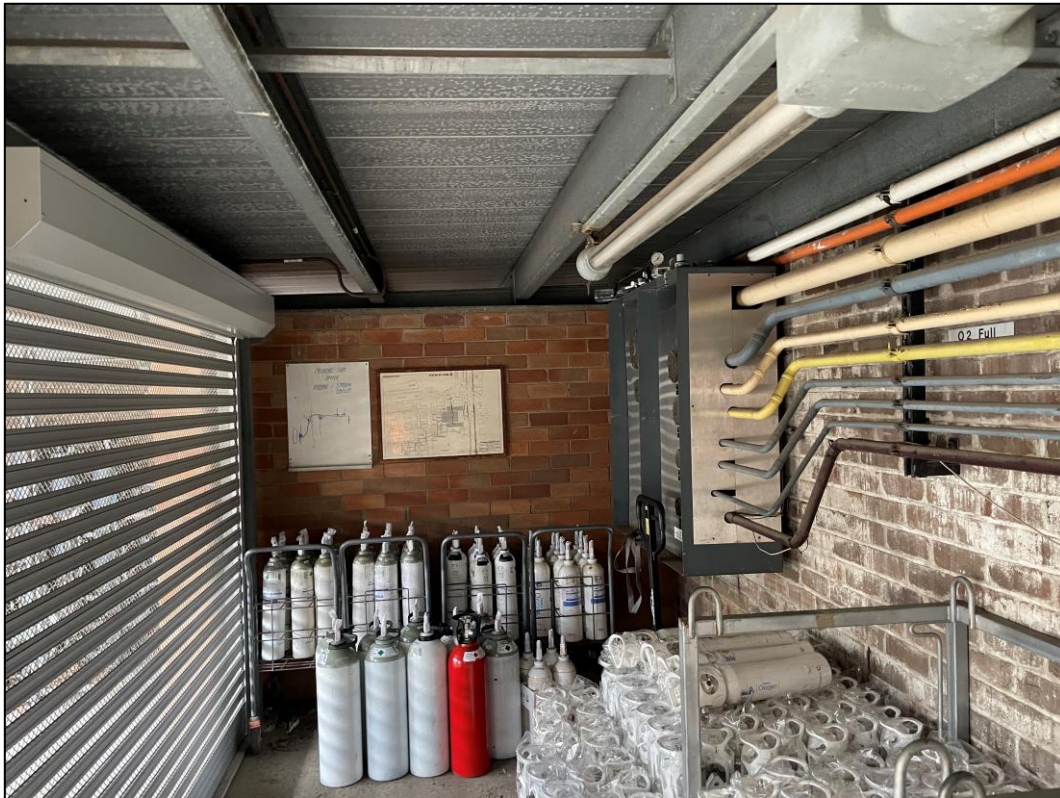
Photograph 3 Example of internal medical gas storage area.
